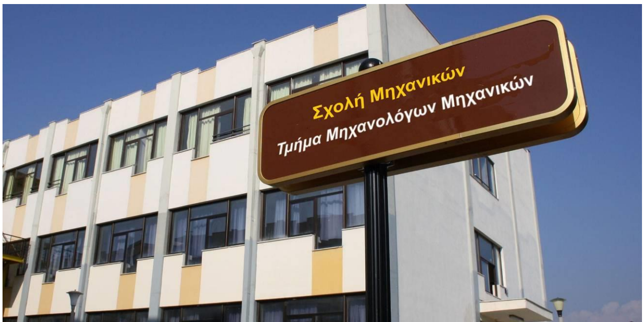
Figure 3. View of the Department's building
